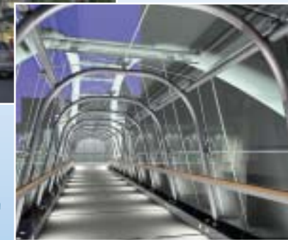
ABOVE: The steel tubing for the main arches is HSS 406mm x 13mm (16" x 1/2") AESS with longitudinal tie rods of HSS 219mm x 6.5mm (8-1/2" x 1/4") AESS.
