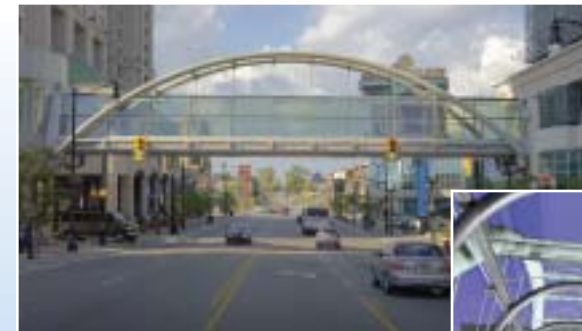
ABOVE: The steel tubing for the main arches is HSS 406mm x 13mm (16" x 1/2") AESS with longitudinal tie rods of HSS 219mm x 6.5mm (8-1/2" x 1/4") AESS.
