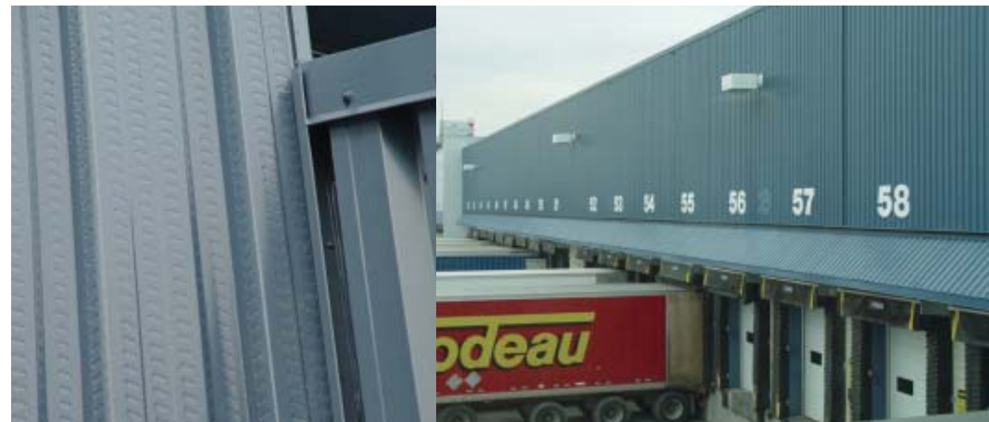
ABOVE: The architecturally integrated prepainted galvanized or Galvalume™ steel Solarwall® system forms part of the buildings fabric.
