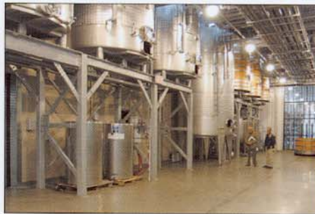
Alan Greer, Sandwell Project Engineer and Adrian Pembroke, Newman Brothers Ltd. on main production floor.
