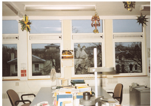
Figure 1 Interior of an office showing trickle ventilators installed in the window frames
