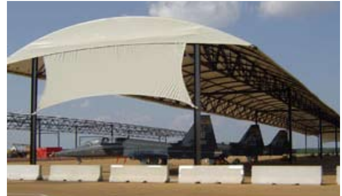
Fig. 10 temporary government shelter
