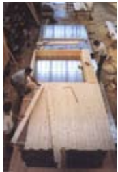
Fig. 28 off-site construction of panels
