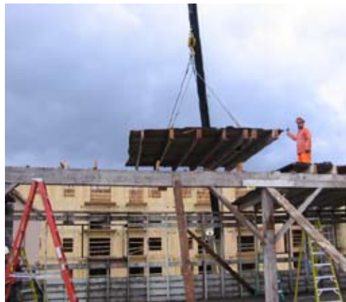
Fig. 13 panelization of roof structure
