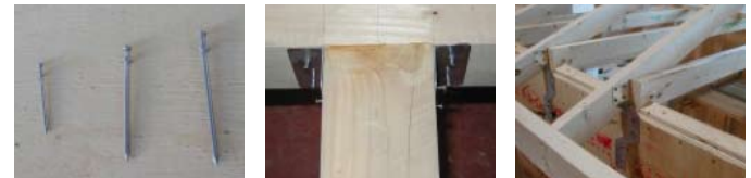
Fig. 11 the double-headed nail in conjunction with metal hangers and plates creates a system that is more easily disassembled than traditional construction techniques
