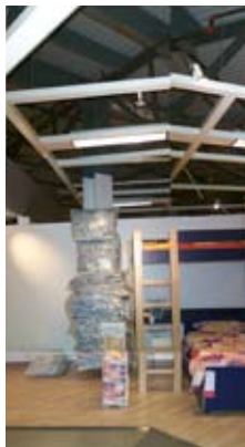
Fig. 51 ceiling grid and partial height display walls
