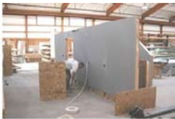
Fig. 34 preassembly of an interior wall
