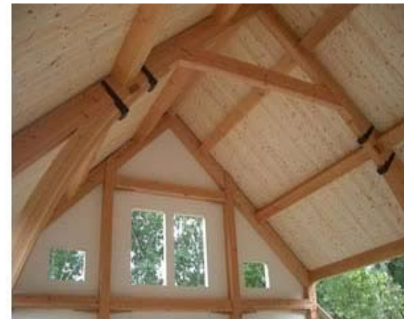
Fig. 36 typical Bensonwood heavy timber framing
