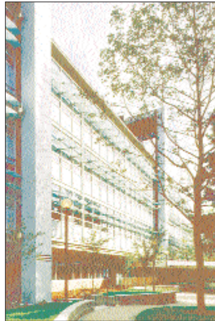
The view from the garden (above) shows ventilation towers and sunshades. A night shot (below) shows a building entry easily accessible from the street or parking area, and (bottom) an interior detail.
