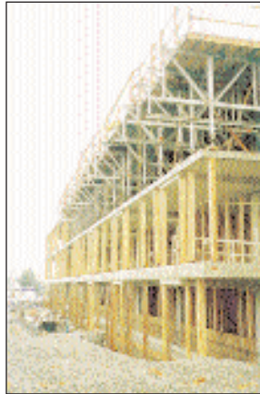
Above: An early construction stage view of the structure
