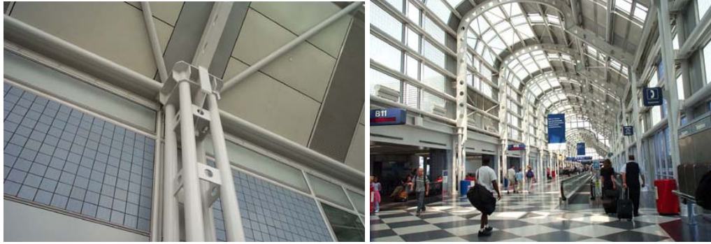
Figures 3 and 4: Interior detail and view of Chicago O'Hare United Airlines Terminal showing the use of architecturally exposed steel structure and high level of transparency.
