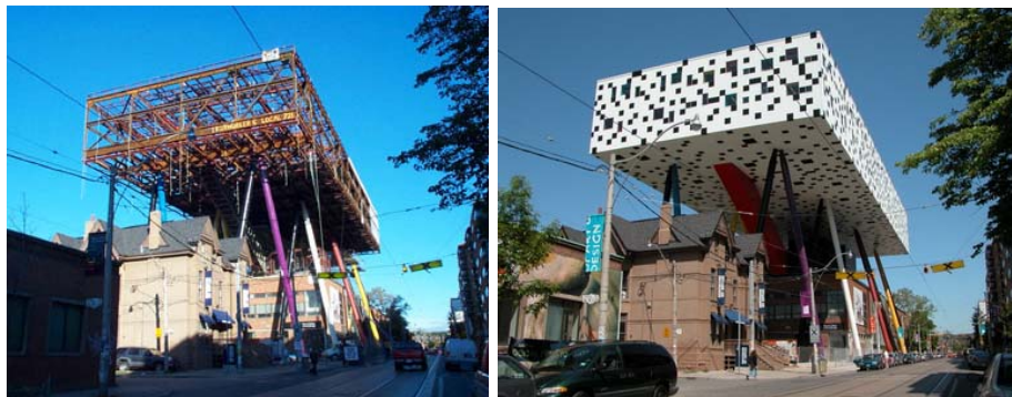
Figures 28 and 29: OCAD Addition, Toronto. During and after construction.
