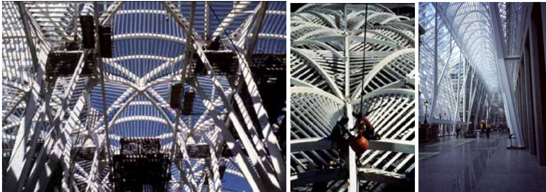
Figures 30, 31 and 32: BCE Place, construction and finished images. Excerpted from SSEF Case Studies CD-ROM Volume 1.
