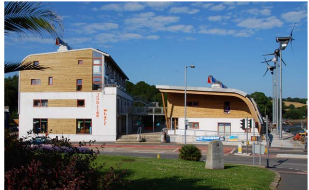
Fig. 4: Jubilee Wharf, Penryn, England – this zero energy development uses 4 micro turbines to provide power. Evacuated tubes provide solar hot water. Roof area for PV has been designed, but no PV is presently installed. Directional wind cowls assist with natural ventilation to the point that no A/C is provided. A 75kW wood pellet boiler provides under floor radiant heating. The building is super insulated with 300mm of insulation netting a U value of 0.1\text{W}/\text{m}^2/\text{°k} . Designed by ZEDFactory. 5
