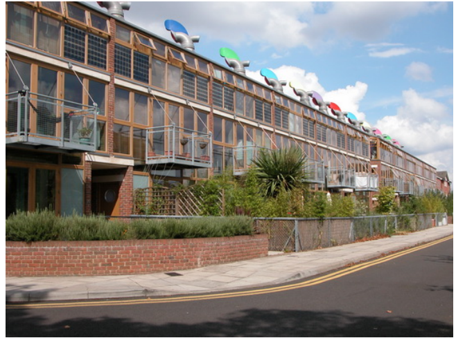
Fig. 2: Beddington Zero Energy Development (BEDZed), Hackbridge, England – the buildings are massed, oriented, glazed and ventilated to maximize their passive potential. Bioclimatic responses to the heating and cooling requirements for buildings will also result in a re-examination of insulation levels and wall construction. In cool to cold climates this infers increasing insulation levels and airtightness in construction. Cold climate buildings that are currently seeking carbon neutrality are working with R values in the floor, walls and ceiling of R30, R40 and R50 respectively. This is a significant increase over current code required levels that require no floor insulation and values of R20 for walls and R30 for ceilings for the same climate severity. 4
