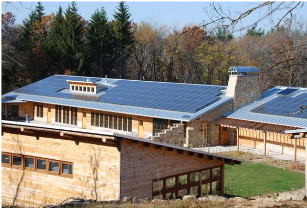
Fig. 3: The budget and resultant square footage of PV was determined at the early stages of design for the Aldo Leopold Legacy Center, and the building was sized to suit.
