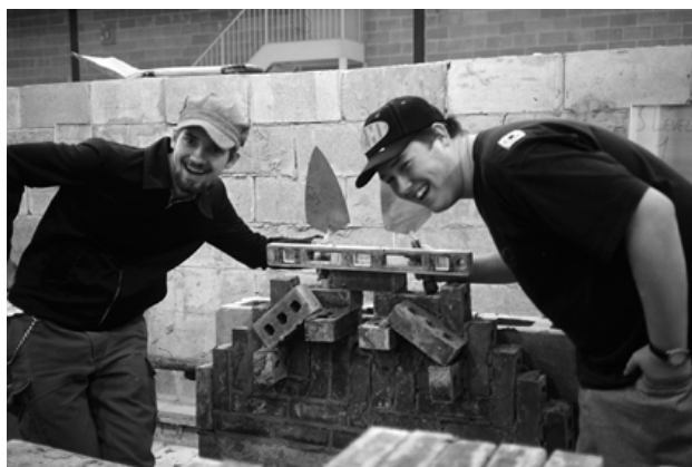
Figure 2: Students Paul Kulig and Matthew Hessey complete a sample masonry cavity wall
