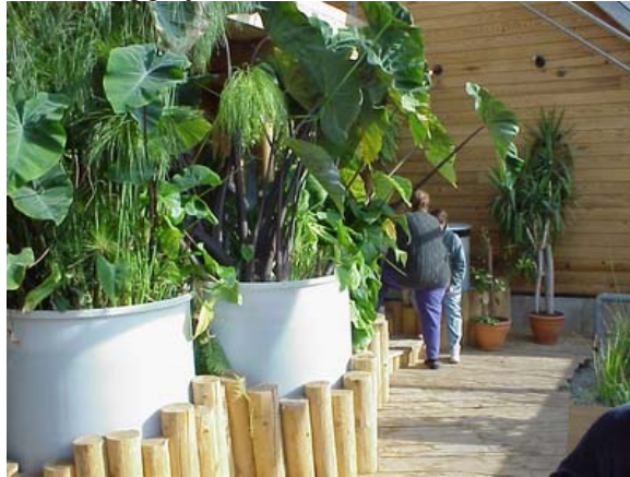
Figure 3: YMCA Environmental Learning Centre, Charles Simon Architect Water Efficiency: Credit 2 Innovative Wastewater Technologies: Living Machine™
