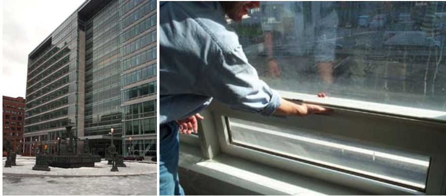
Figure 7: Innovation and Design Process: Caisse de Depots et Placements, Montreal Double skin wall construction.
