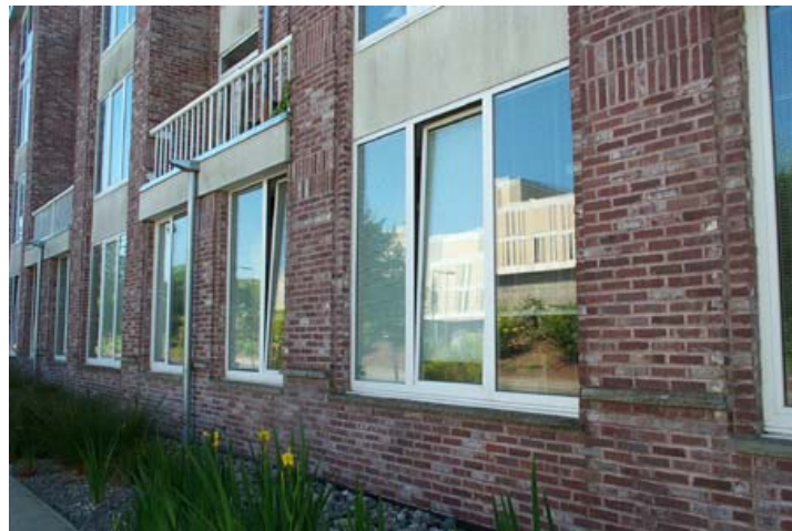
Figure 6: C.K. Choi Institute for Asian Studies, UBC, Matsuaki Wright Architects Indoor Environmental Quality: Ventilation Effectiveness + Control of Perimeter systems
