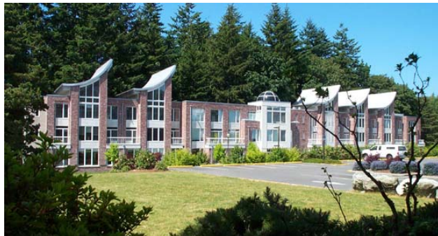
Figure 5: C.K. Choi Institute for Asian Studies, UBC, Matsuaki Wright Architects Materials and Resources: Credit 4 Recycled Content (both the timber frame and brick veneer cladding)
