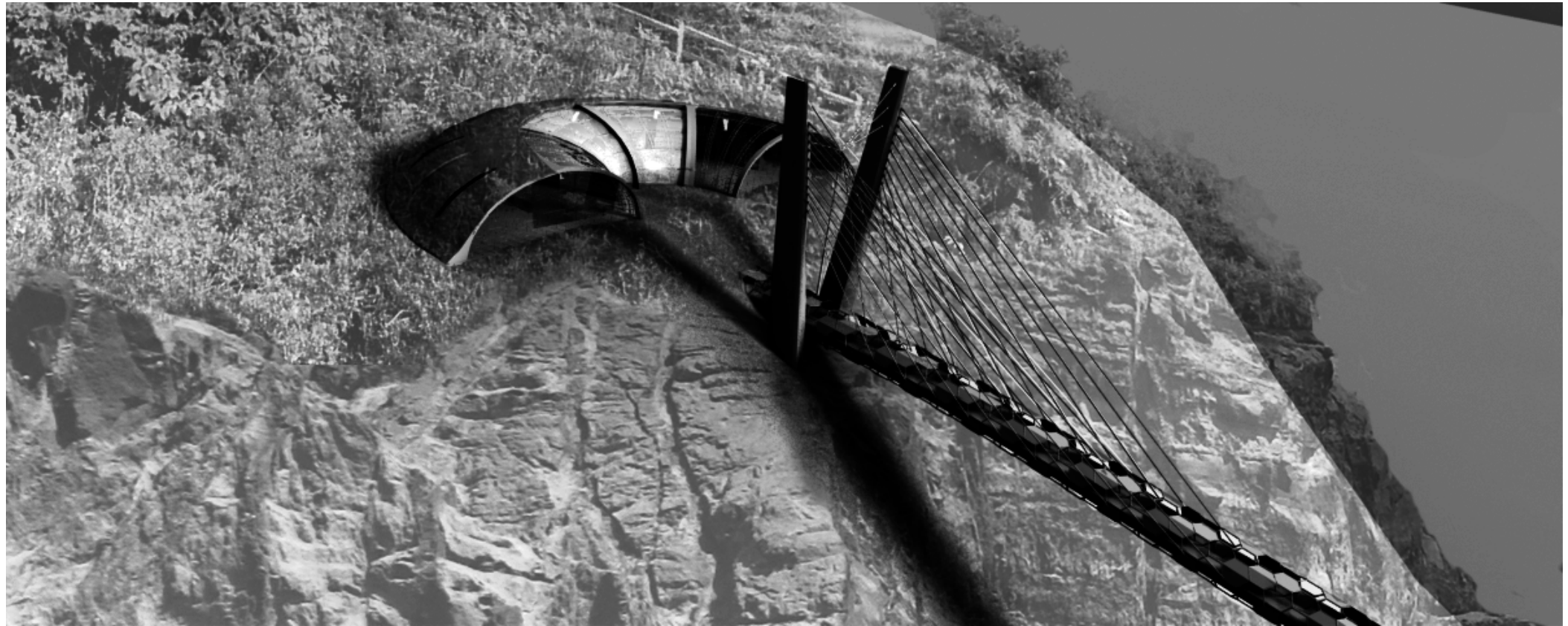
VIEW OF THE DIOMEDE BRIDGE EXITING FROM THE CLIFF OF BIG DIOMEDE ISLAND
