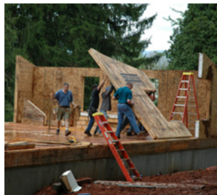
installing SIP panels
