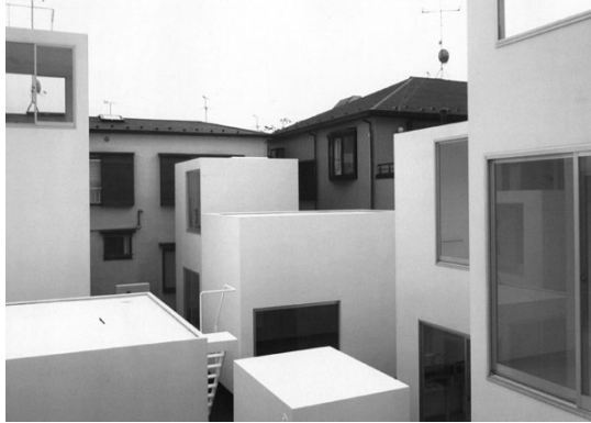
5 Moriama House, The Office of Ryue Nishizawa
