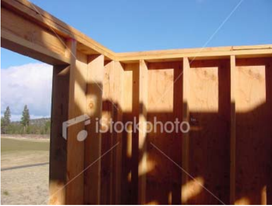
Wood stud wall with plywood shear panels
