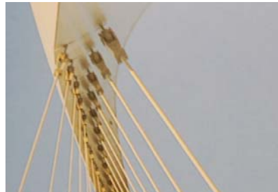
Tensile joint by Santiago Calatrava
