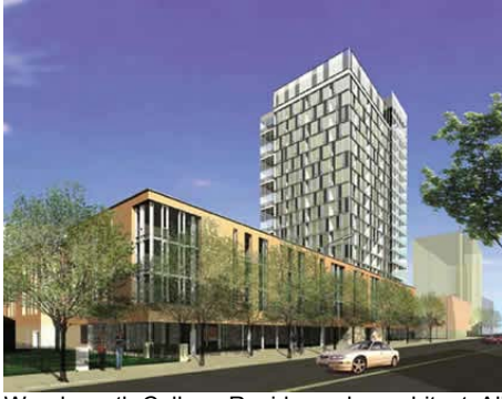
Woodsworth College Residence by architectsAlliance
