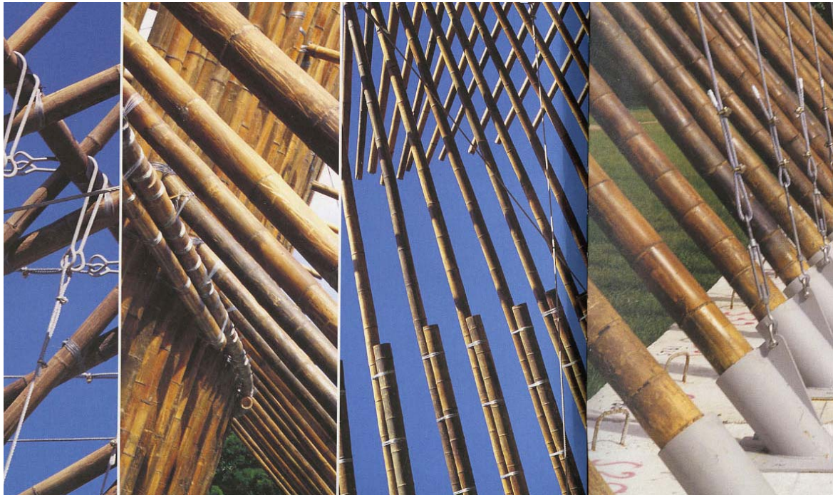
Figure 20 Steel Cable Reinforcing and Connections (Gutierrez, 32)
