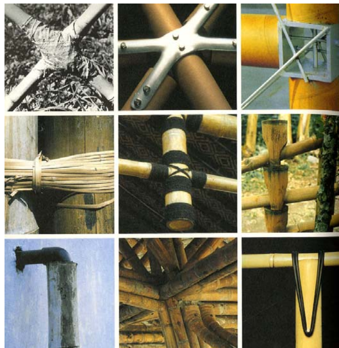
Figure 21 Other Bamboo Connections (Kries, 114)
