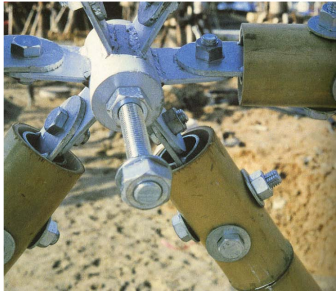
Figure 9 Bamboo Connection (Kries, 108)
