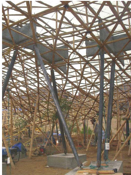
Figure 13 The Mexican Roof - Flattened Bamboo Structure (Prix, 59)
