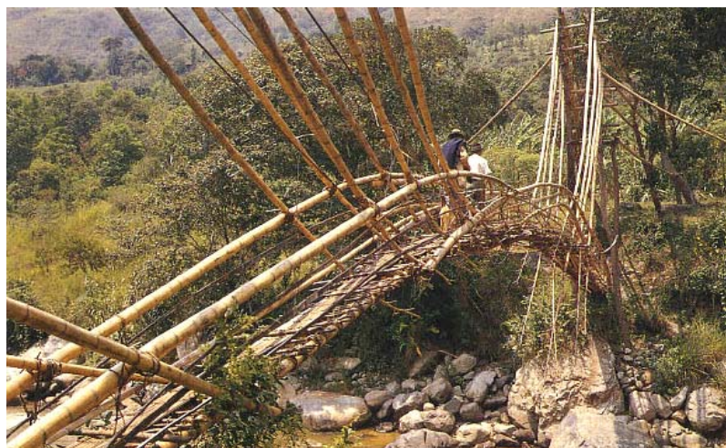
Figure 7 Bamboo Bridge (Villegas, 23)
