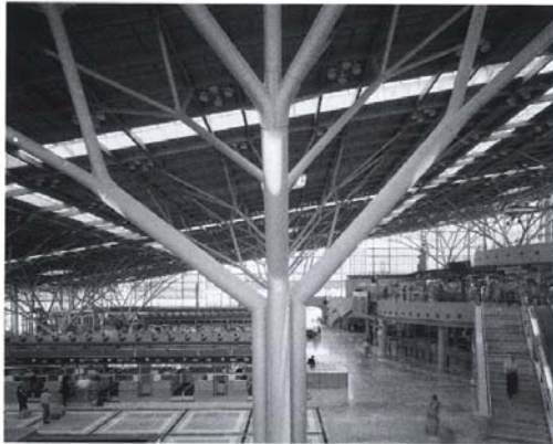
1.12 Stuttgart Airport Roof using tubular column 'trees' — see also Colour Plate 9 (architect: Von Gerkan Marg & Partners)
