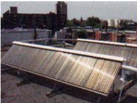
Figure 7 Evacuated tubular solar collectors
