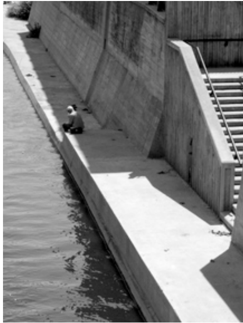
Figure 3: West wall of the levee
