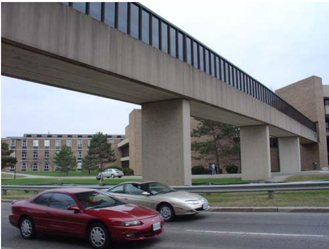
Existing pedestrian bridge at the University of Waterloo
