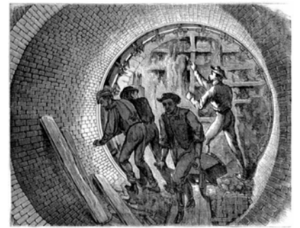
Digging the Beach Pneumatic tube with the shield. From Scientific American, March 5, 1870.
