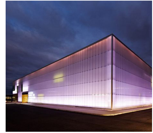
fig08 polycarbonate facade precedent
