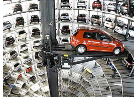
fig05 automated car garage
