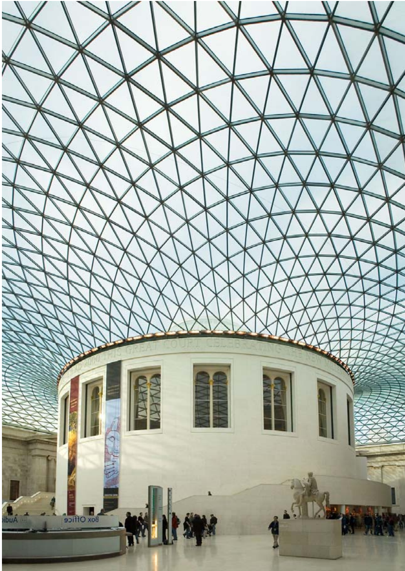
British Museum Great Court Roof by Foster + Partners 6
