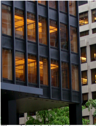
The ordained shading devices proved to be a useful precedent in designing the façade [1]
