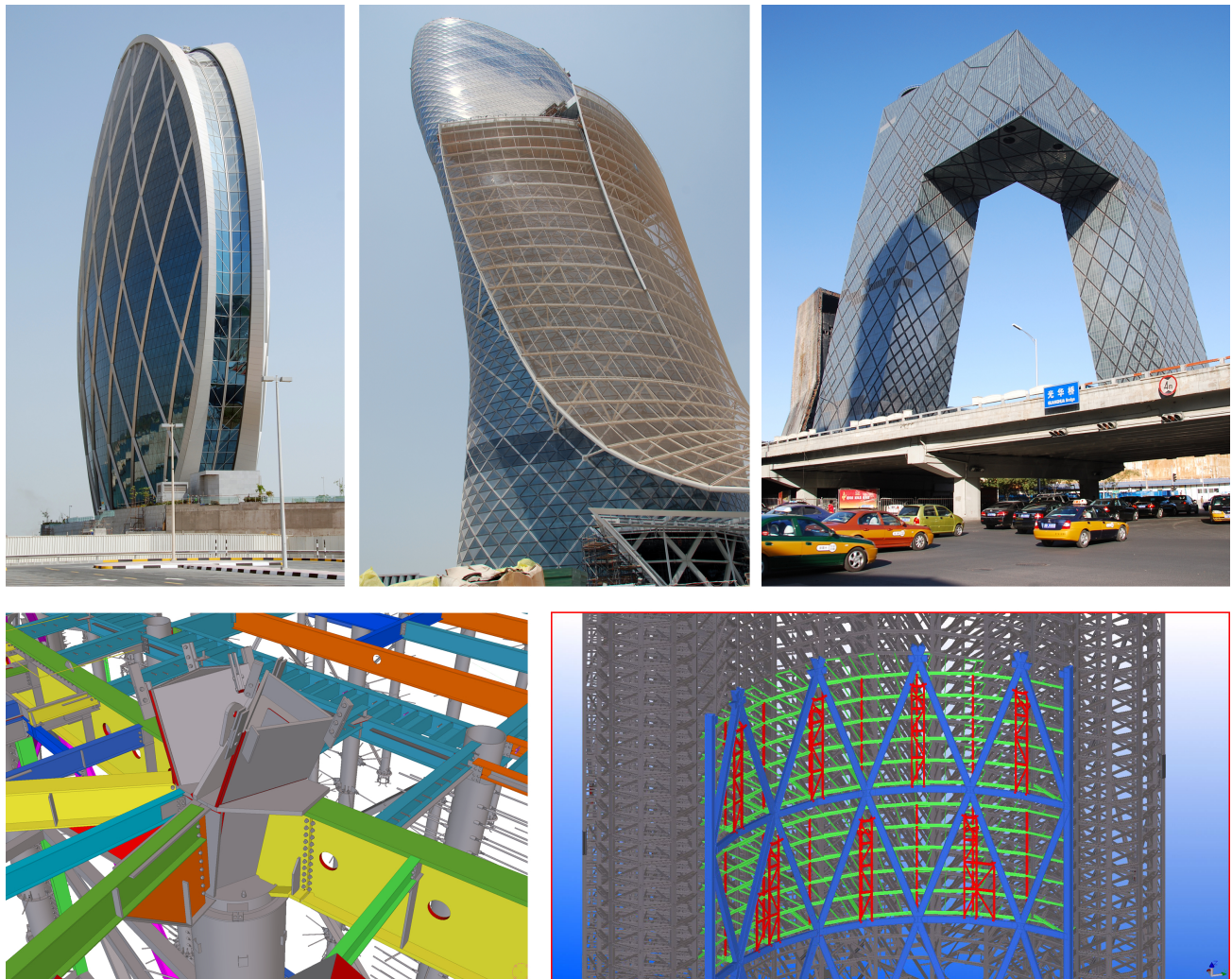
Figure 5. Aldar Headquarters in Abu Dhabi (2010)(top left) uses a diagrid to create the only circular tower (in elevation) in the world. Capital Gate in Dubai (2011) (top middle) is the most backwards leaning tower. At 18^\circ its lean exceeds that of the Leaning Tower of Pisa. CCTV in Beijing (2010)(top right) is strictly speaking not a pure diagrid tower as it also relies on vertical columns for support. But the diagrid was essential in constructing the remarkable cantilevered sections without aid of shoring. 22 The digital images created by the fabricator 23 for the Bow Encana in Calgary, AB, Canada reveal the complexity of the construction of a diagrid node (bottom left) as well as the staging and shoring for the installation of the long diagonals (bottom right). Erection in eccentrically loaded diagrid buildings is far more difficult than in more historic orthographic towers.
