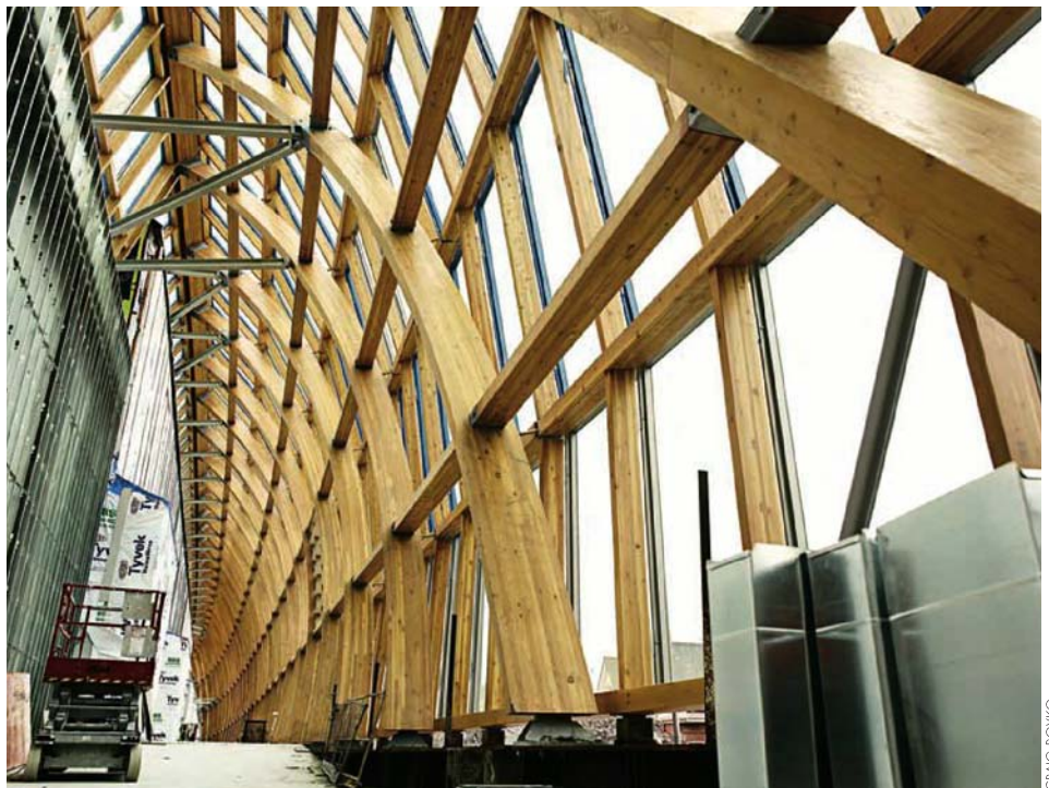
TOP A VIEW OF THE UNDERSIDE OF ONE OF THE CURVING STAIRCASES REVEALS THE COMPLEX DESIGN OF ITS STEEL STRUCTURE. MIDDLE LEFT THE STAIRCASES WERE ALL FABRICATED AND PRE-ASSEMBLED OFF-SITE BY MARIANI METALS. MIDDLE RIGHT THE STAIRCASE AS A DRAMATICALLY EXPRESSED ELEMENT, THRUSTING THROUGH THE BUILDING'S ELEVATION. BOTTOM A VIEW DOWN THE ATRIUM SPACE OF THE NORTH GALLERY. CURVED GLULAM MEMBERS ARC GRACEFULLY OVERHEAD.
