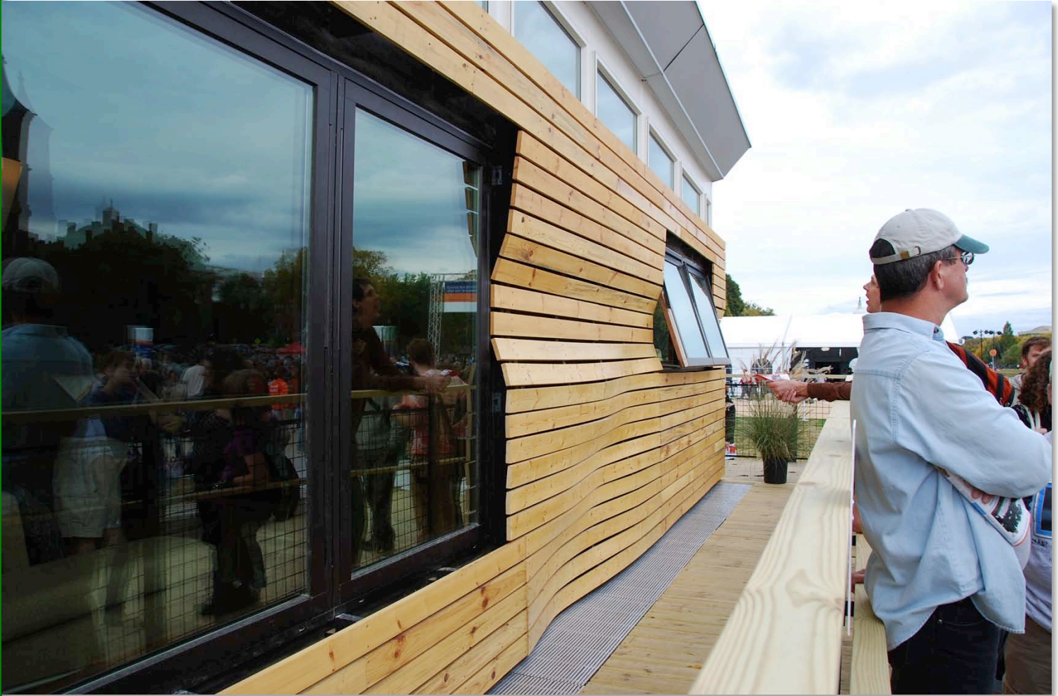
Experimental cladding presents challenges for detailing the building envelope.
