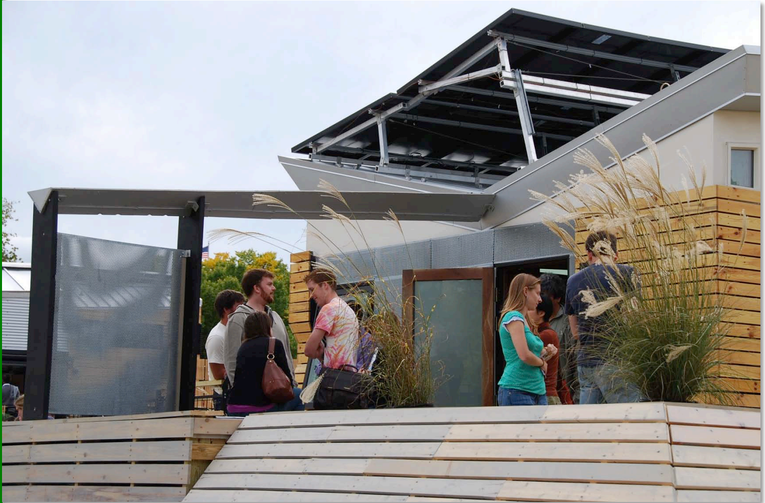
Butterfly roof for water collection presents challenges for detailing the building envelope.
