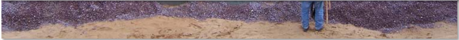
Installation of large earth ducts to preheat and precool the air.
