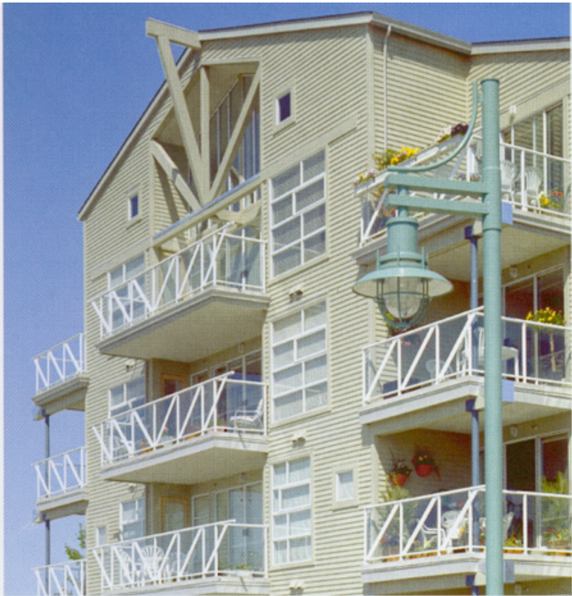
Figure 2 Four Storey Wood Frame Residential Construction
