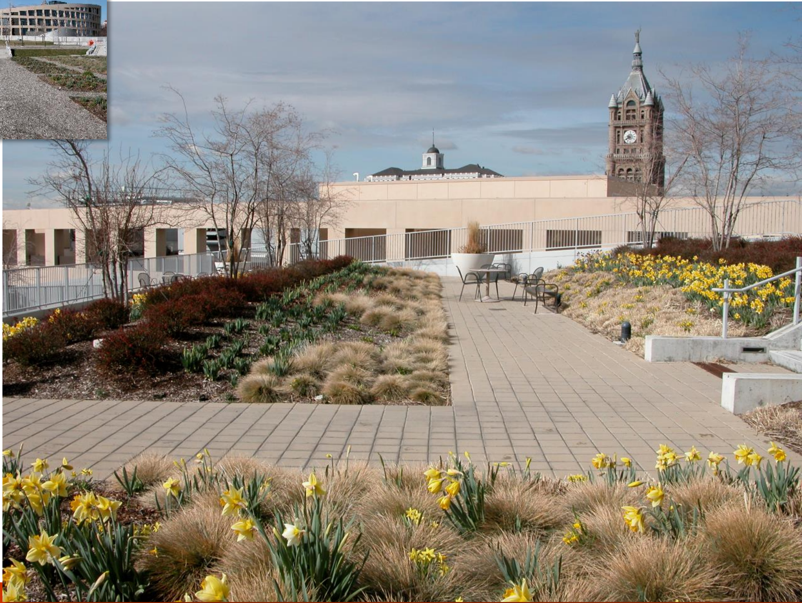
Partial green roof on the Salt Lake City Library by Moshe Safdie
