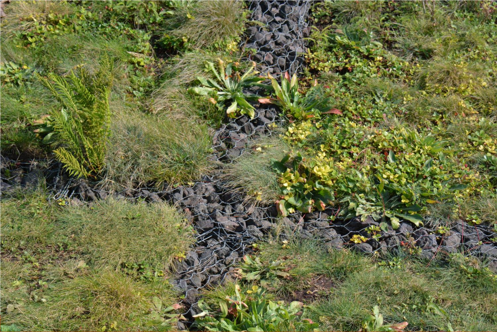
Drainage paths for excess water
