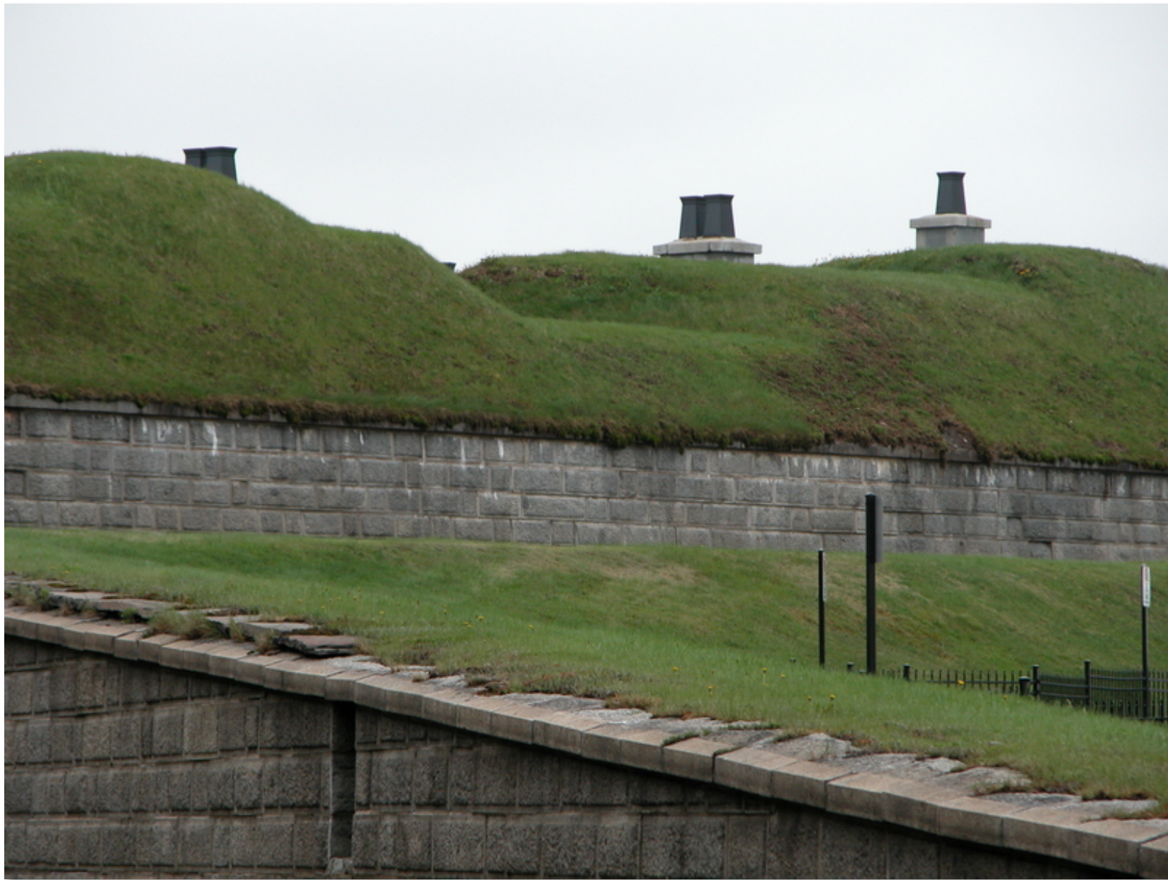
Very old green roof over the Halifax Citadel.
