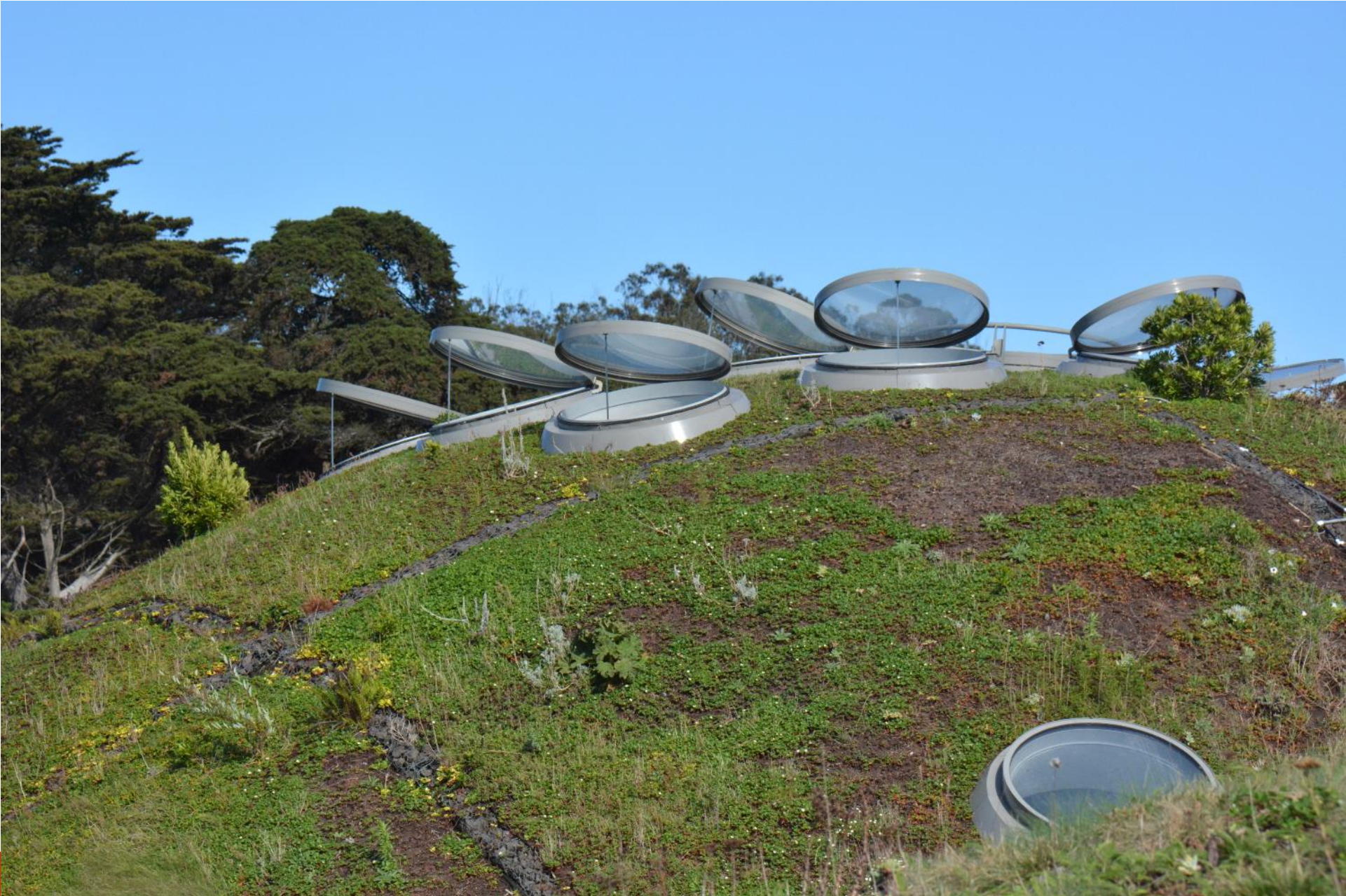
Operable skylights to vent heat from interior
