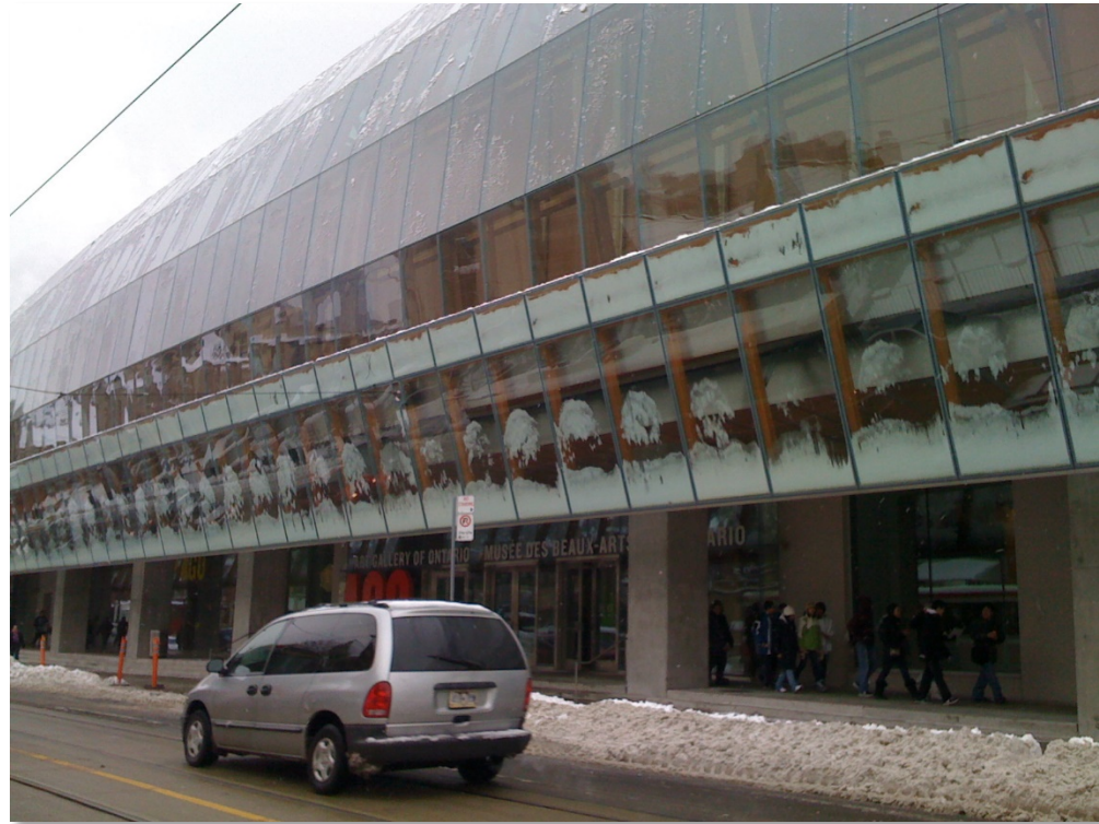
Odd shaped buildings like the AGO by Frank Gehry are not immune to difficult snow accumulation.
