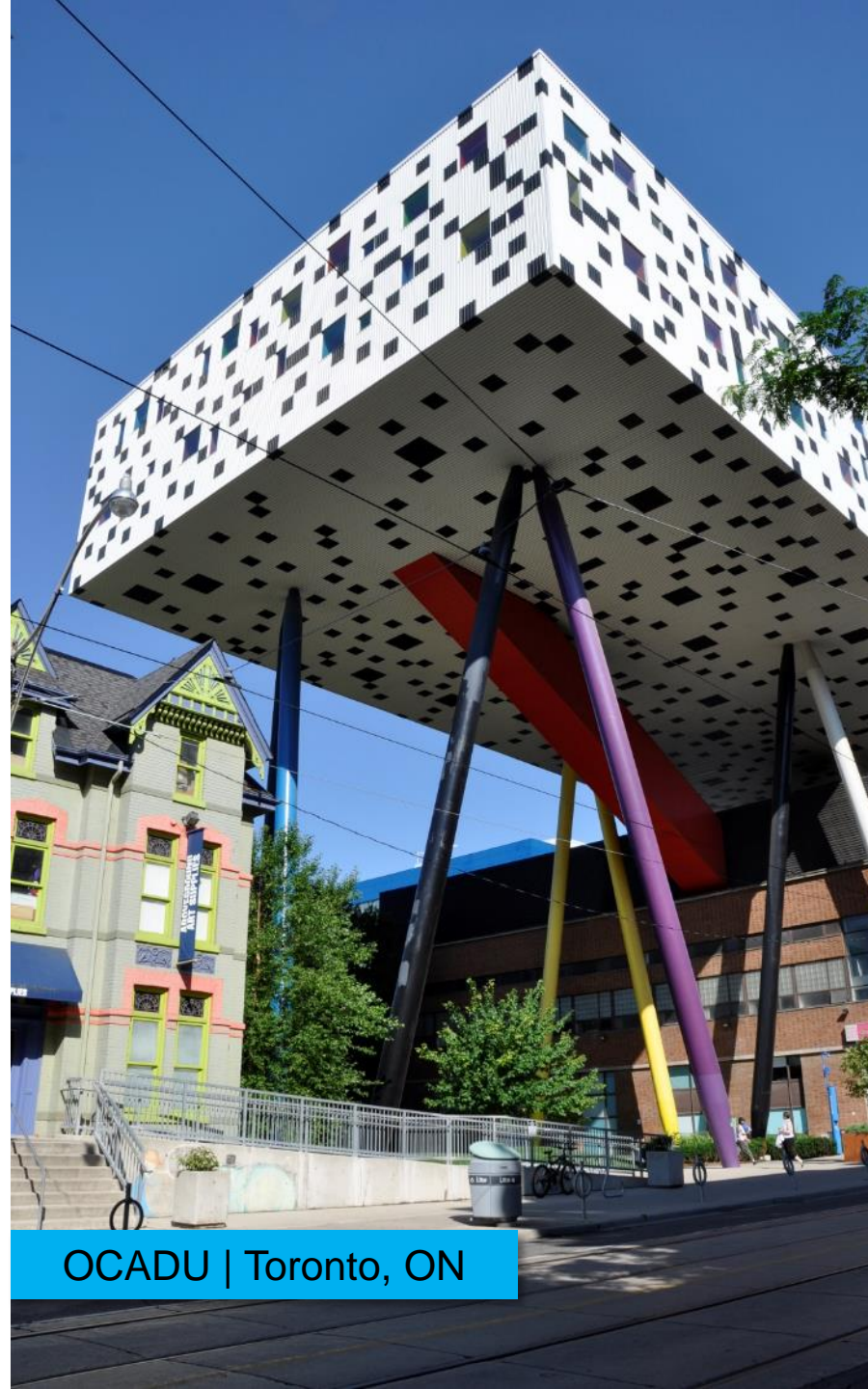
Fabrication and Erection: Walters Inc.
