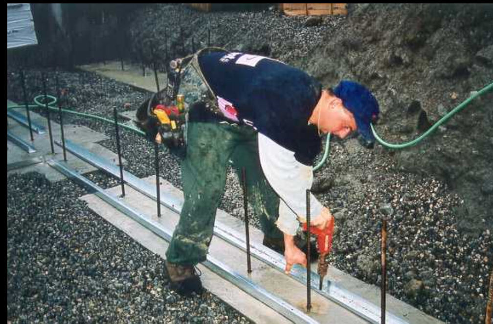
Insulated concrete forms (ICF)
