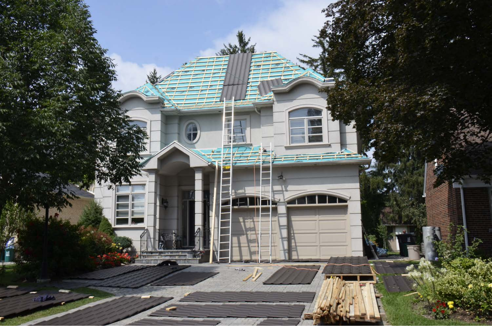
Contemporary tile look roof with underlayment
