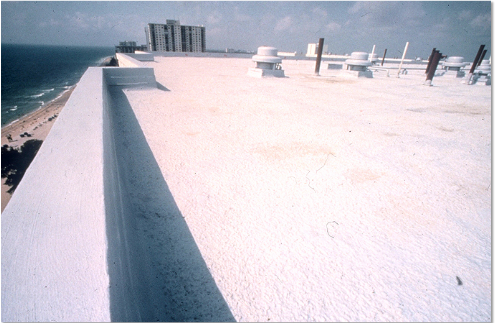
Spray applied elastomeric membrane roofing
