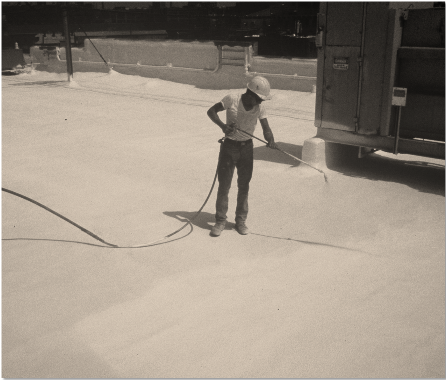
Spray applied elastomeric membrane roofing
