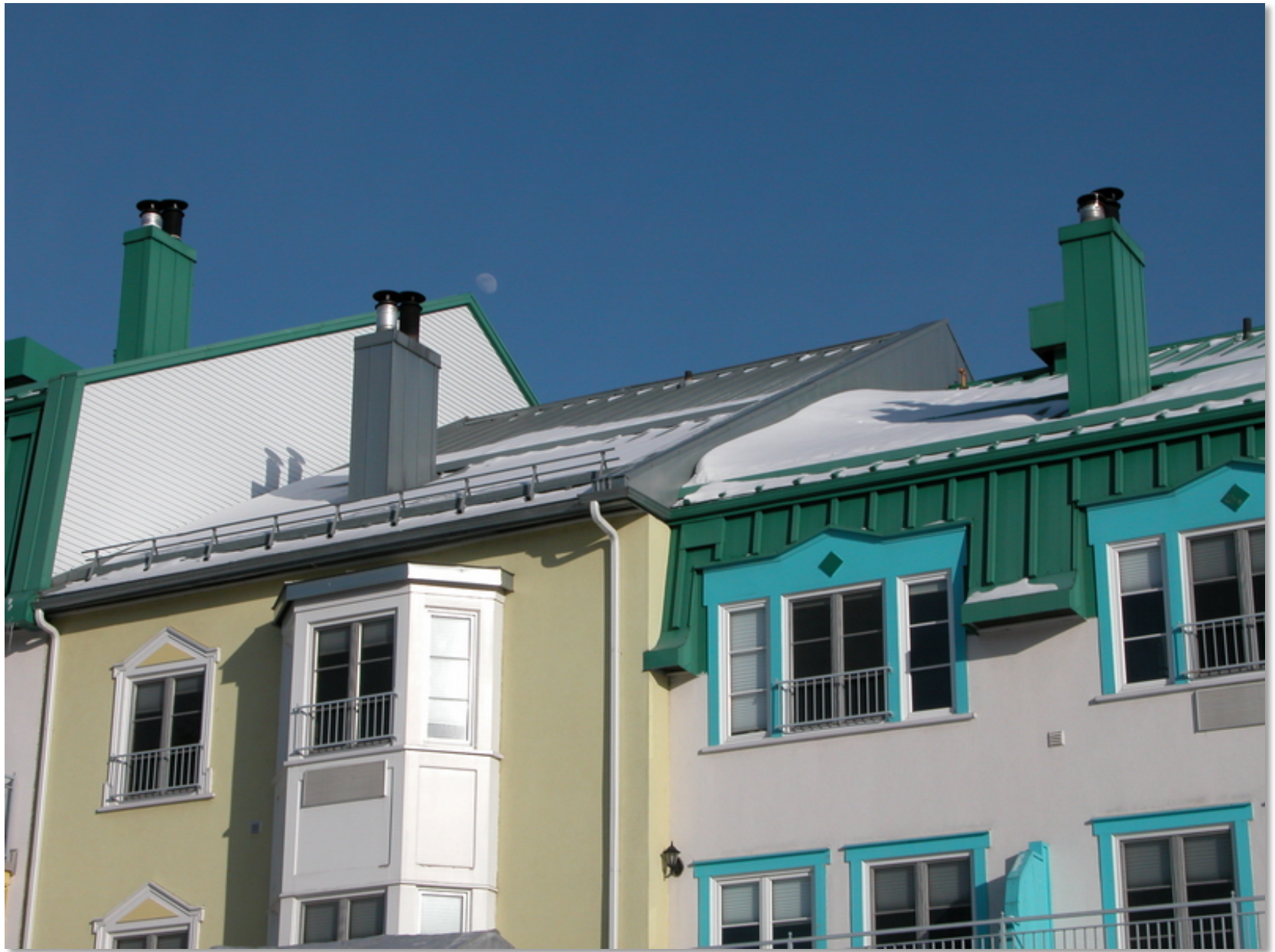
Snow guards at the edge of roofs
