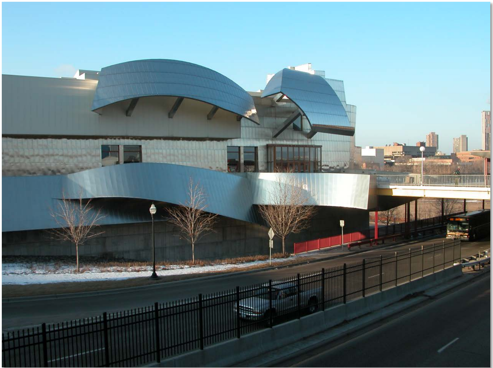
The Gehry Weisman Art Museum in Minneapolis used similar techniques for the stainless steel cladding panels.
