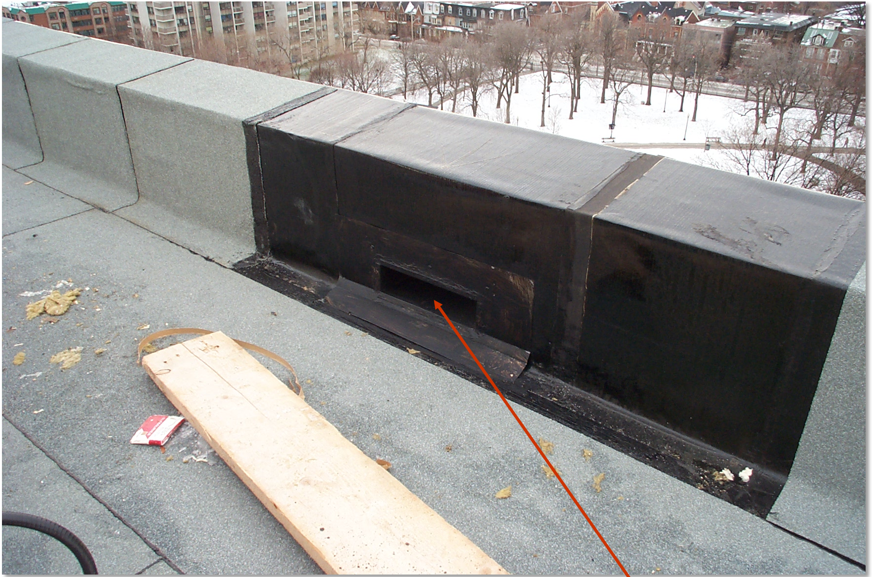
Detail at parapet. Note water overflow opening.
