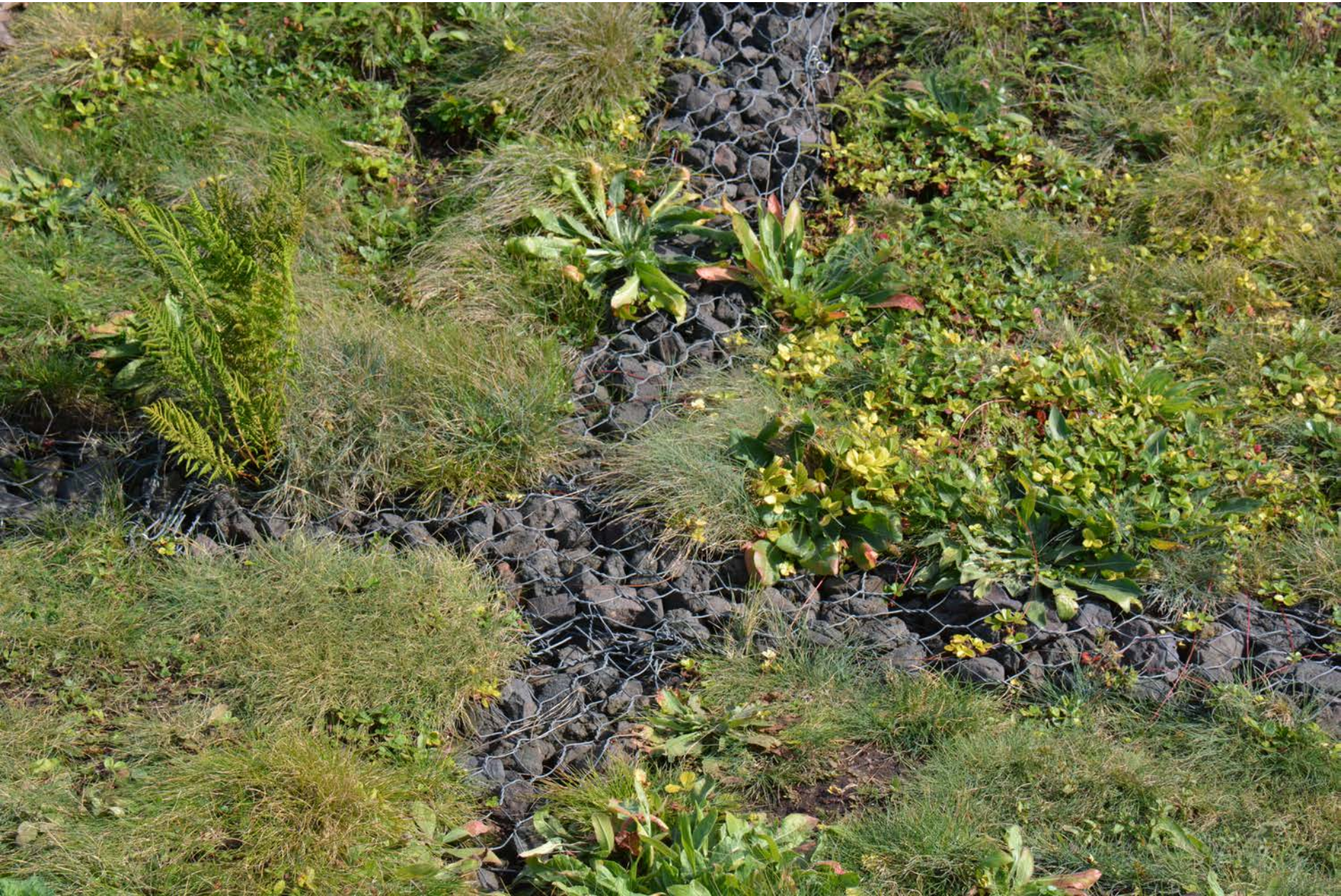
Drainage paths for excess water
