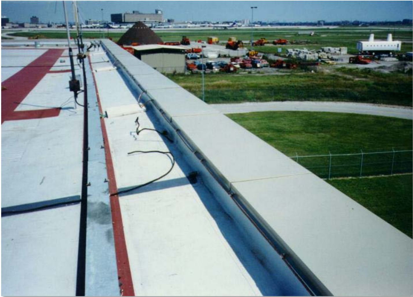
PVC Roof at Pearson International Airport
