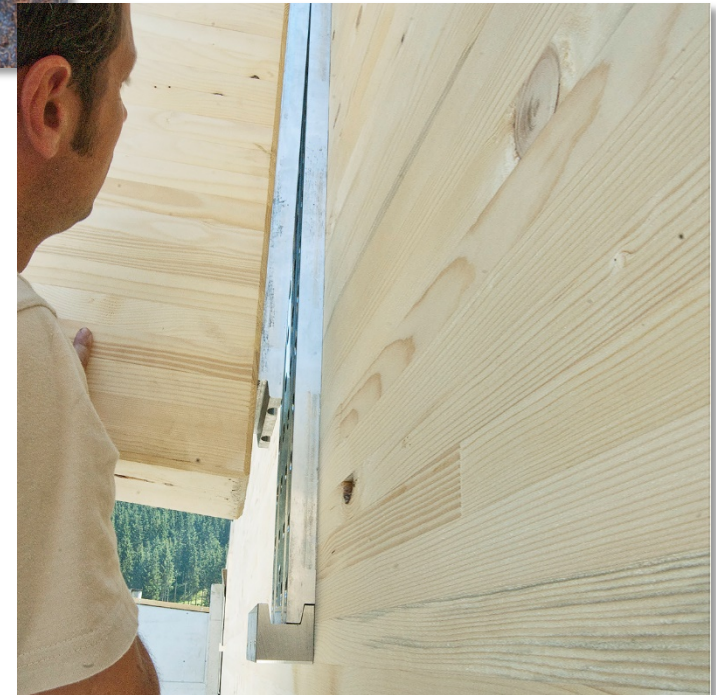
Megant fastener system for beams
