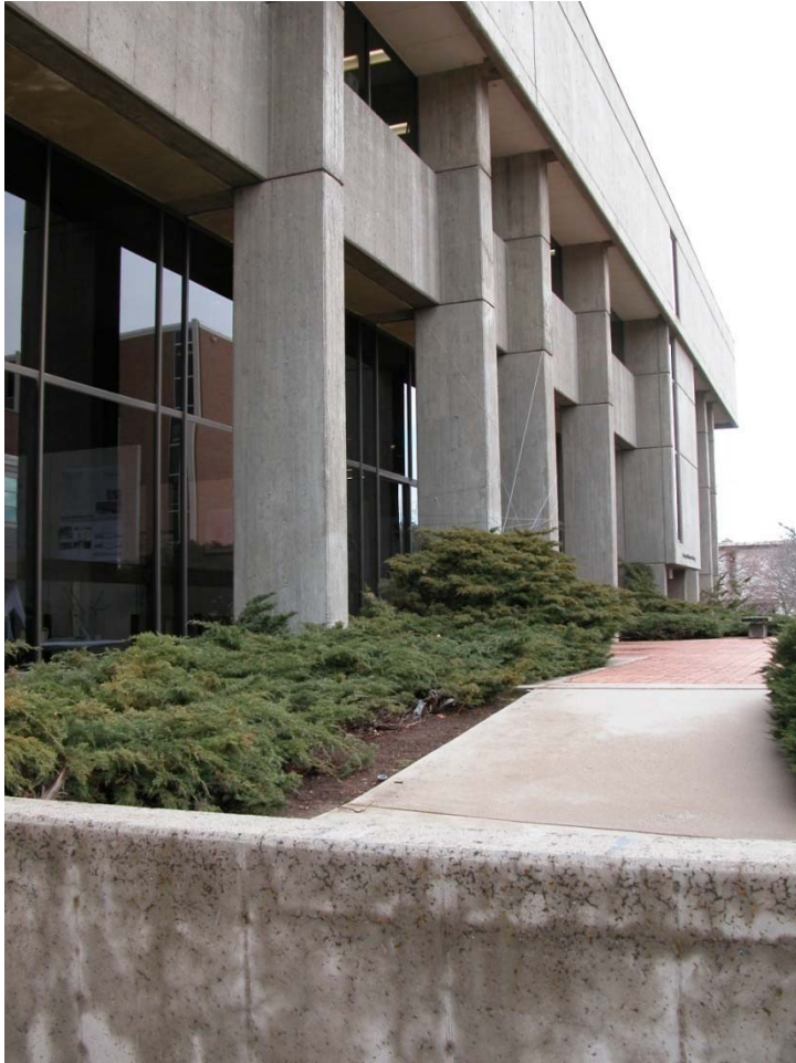
Utah School of Architecture – reinforced concrete
