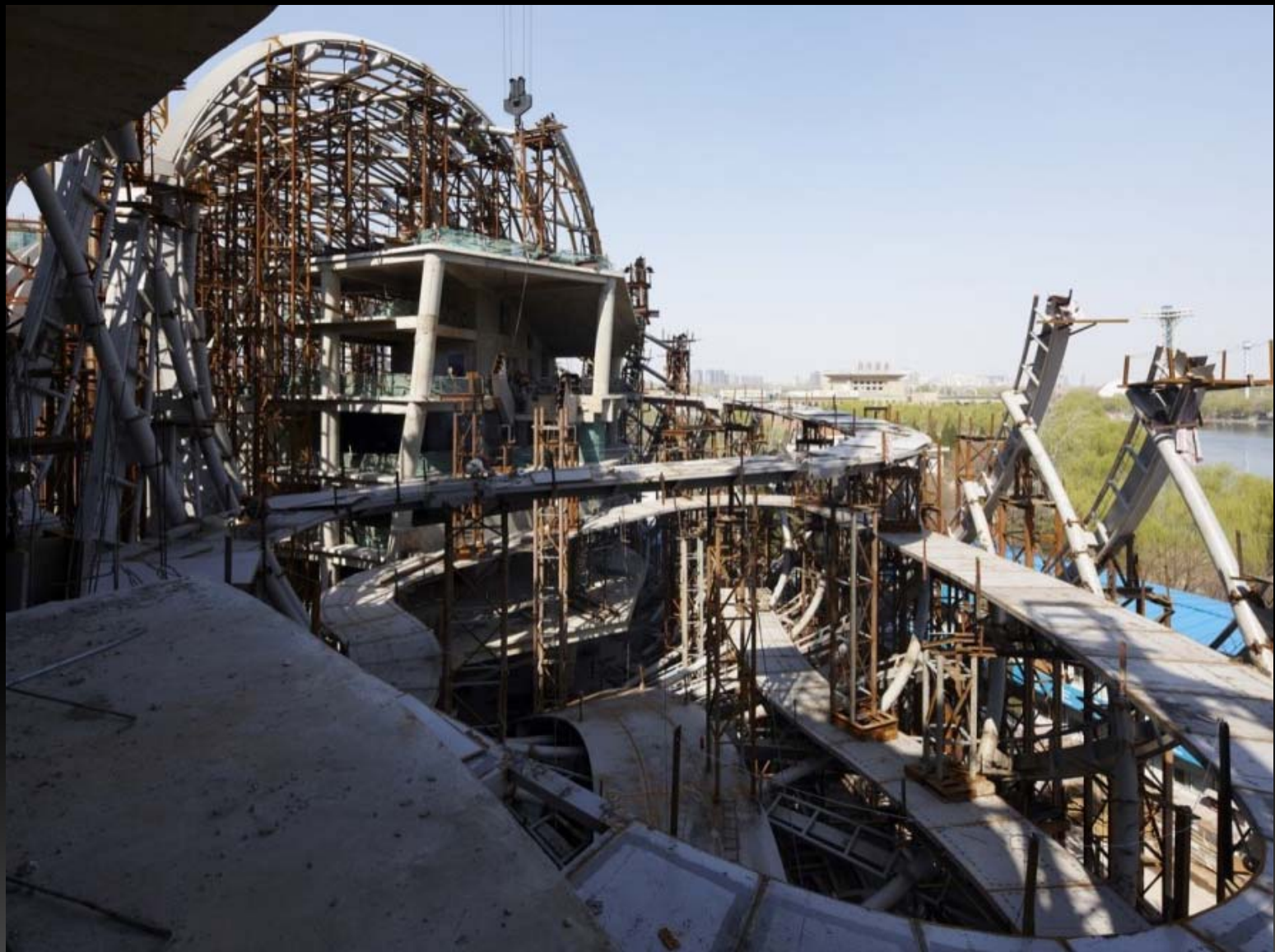
Interior view of construction of spiraling ramp.
