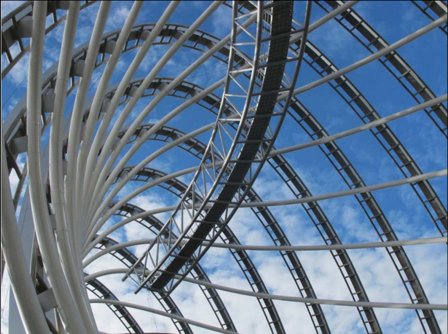
Interior view showing construction of upper spiraling ramp.
