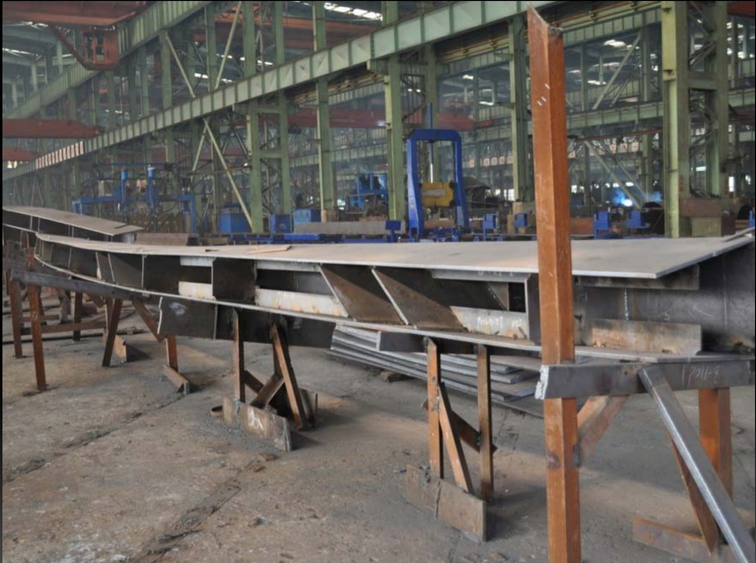
Ribs constructed from custom plate with interior reinforcement.
