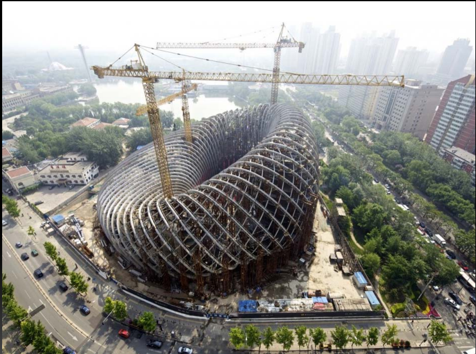
Aerial view during latter stages of construction.
