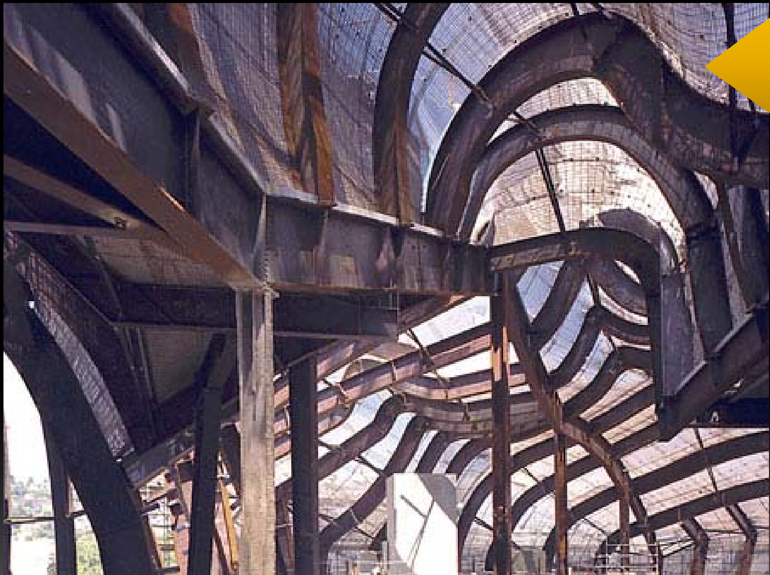
Raw steel frame.
