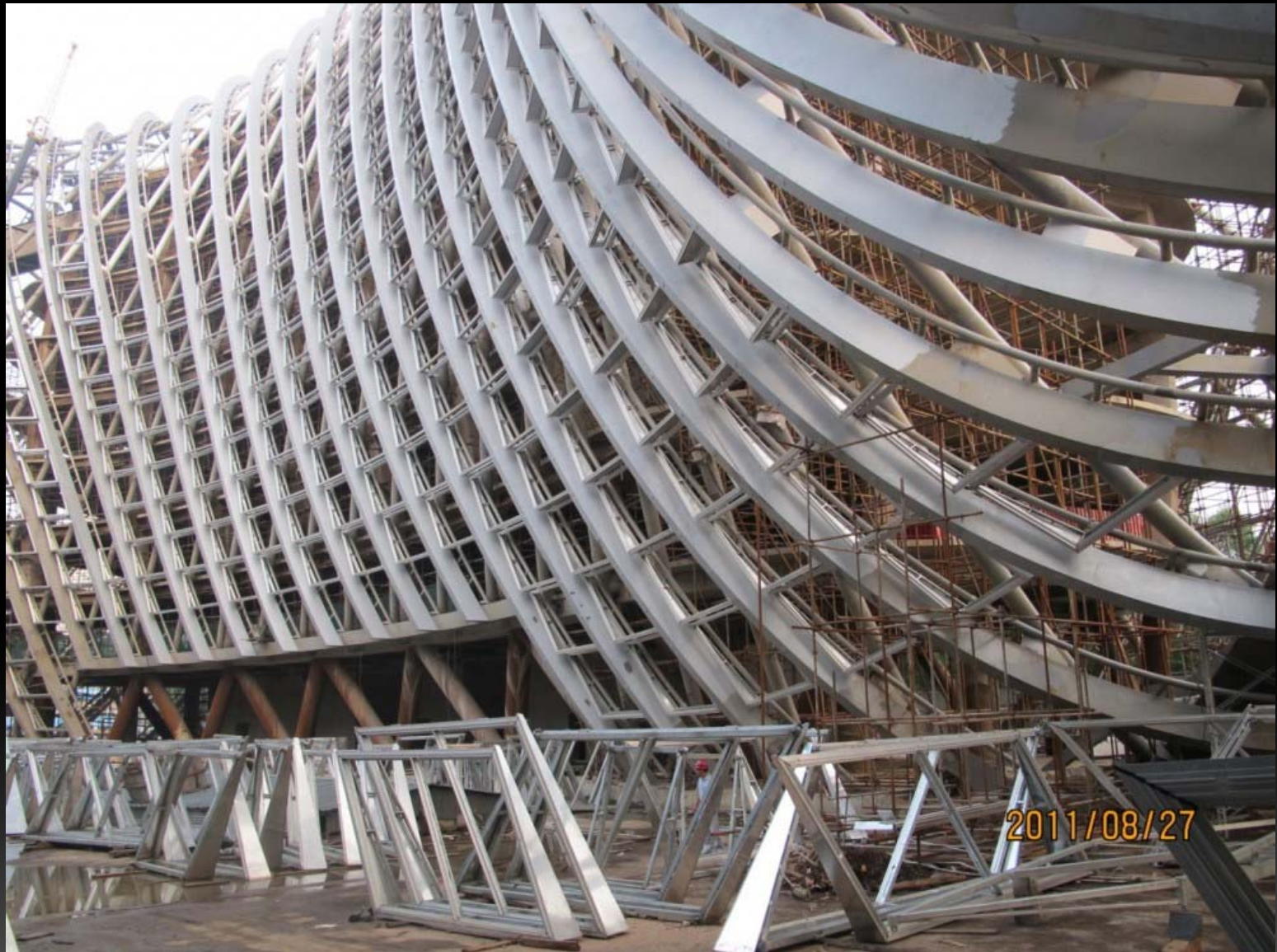
Installation of shingled glazing system.
