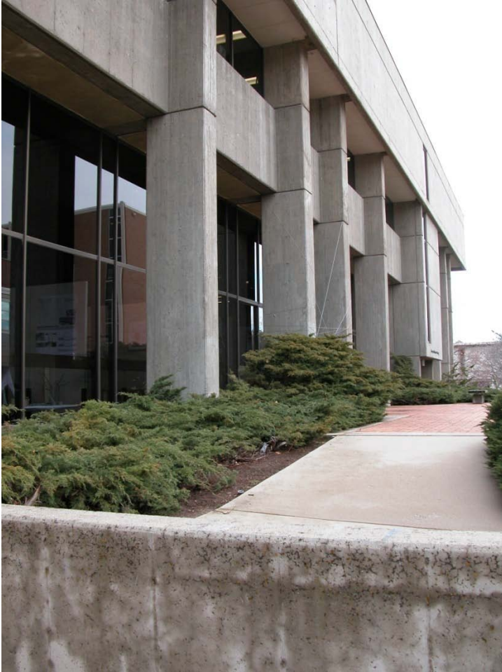
Utah School of Architecture – reinforced concrete
